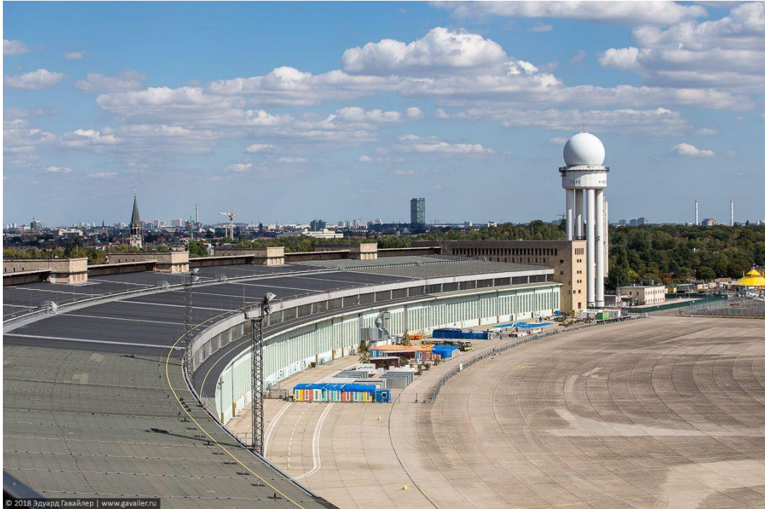
Fig 2.2 View of the airport territory after its completion
